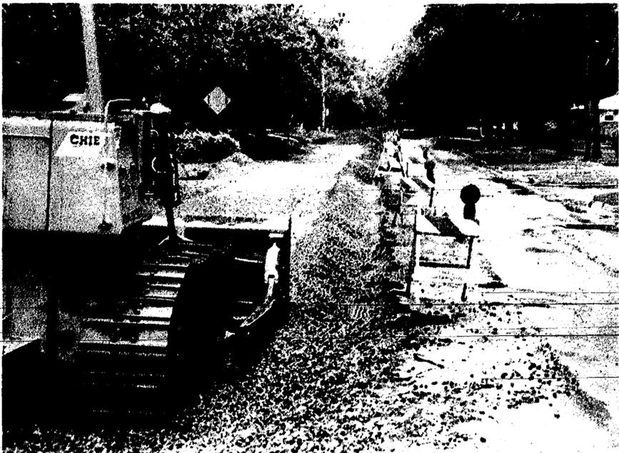
**PAVING OF 950 FEET** of much traveled Wilkinson St. has begun. The paving company is working on one side of the street at a time so traffic won't be cut off completely. However, the situation has created hazardous traffic conditions, so motorists should use extra caution. The work involves repairing the entire road base.
